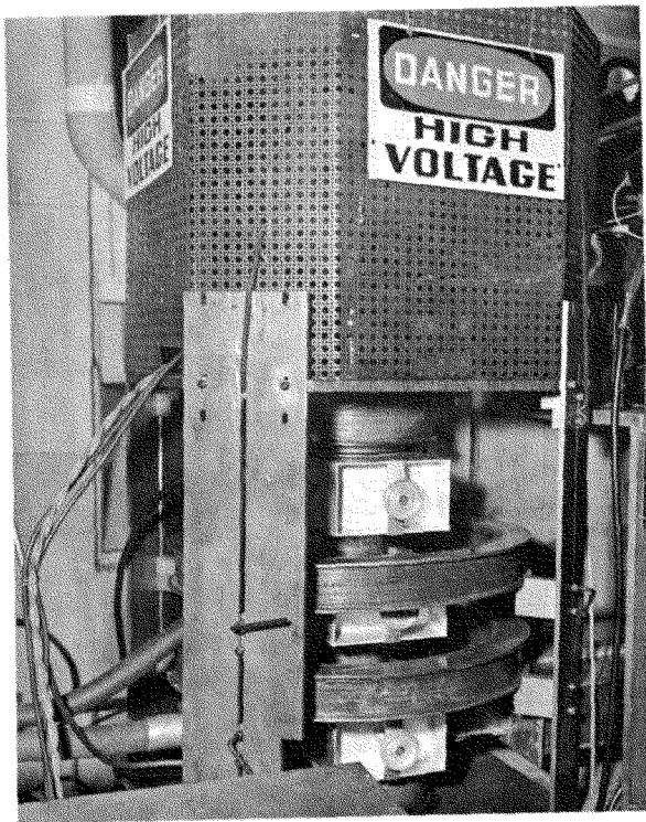
Fig. 8—The 5-kw klystron on test.
